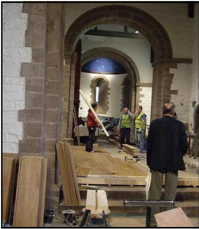
Work underway in St Peter's
